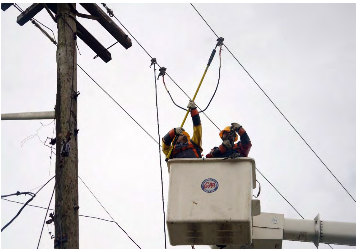
Figure 14: Guam Power Authority Crews restoration efforts well underway
