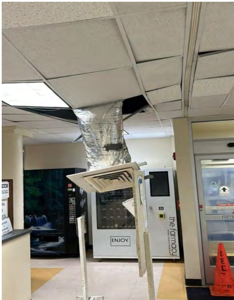
Figure 12: Blown out air-ducts at the Guam Memorial Hospital
